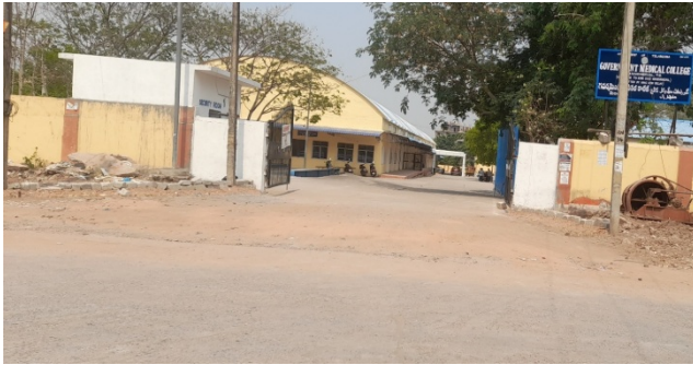
Figure 2. Medical college functioning in a temporary establishment
