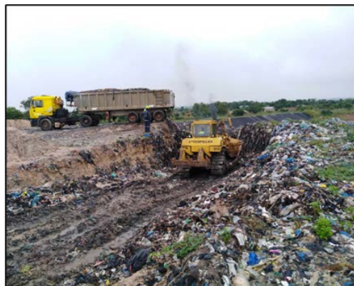
Figure 2. Status of the Technical Landfill Center locker
