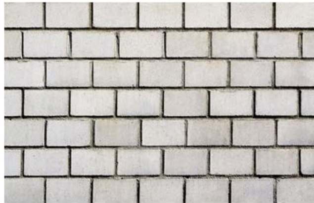
Figure 4. Masonry wall constructed of calcium silicate bricks
