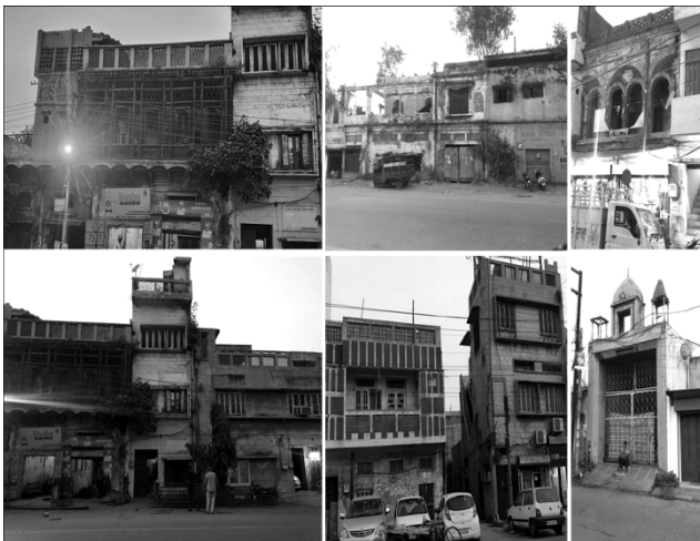
Figure 9. Old structures along the selected road
