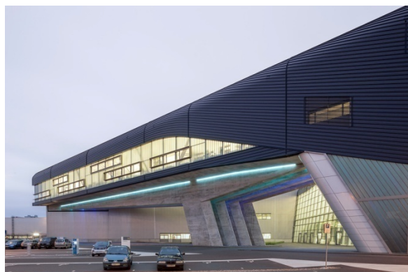
Figure 3. The BMW Central Building at Leipzig, Germany
