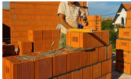
Figure 4. Load bearing Porotherm Clay Brick wall
