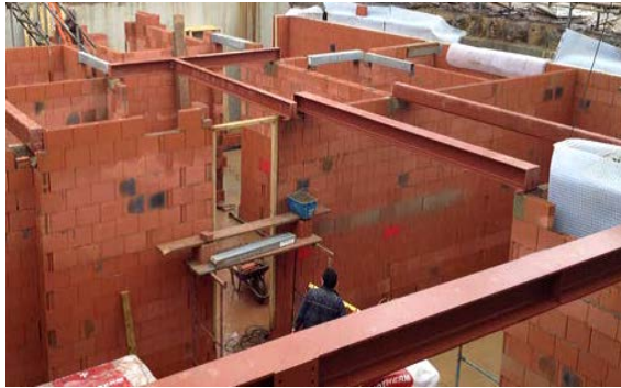
Figure 5. Masonry walls constructed by Porotherm Clay Bricks
