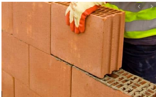
Figure 3. Ease of construction with Porotherm Clay Bricks
