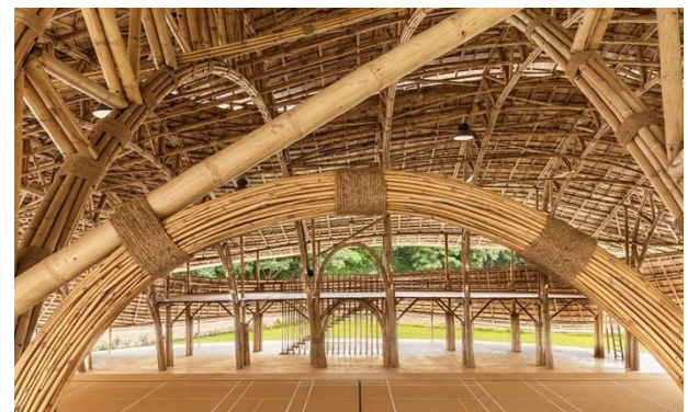
Figure 14. Structural system of Bamboo Sport Hall at Chiang Mai
