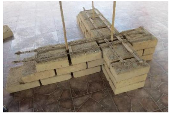
Figure 2. Application of adobe blocks in walling system
