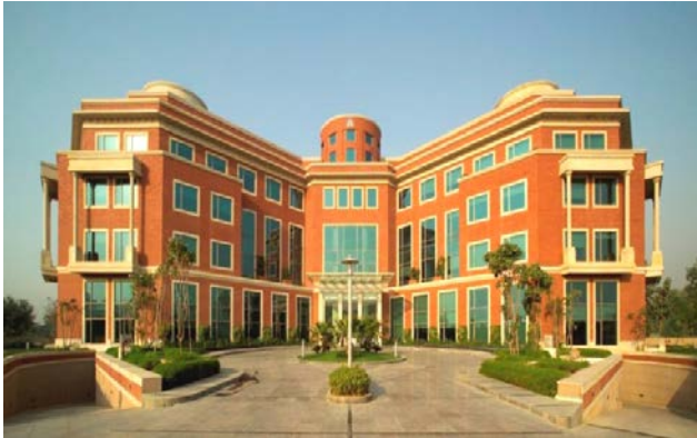
Figure 5. Double glazed windows in ITC Green Centre at Gurugram, India
