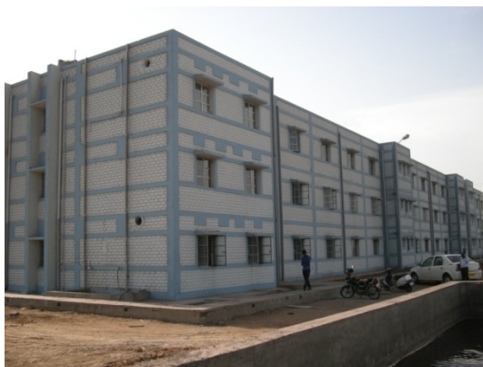
Figure 11. A Three storeyed housing with interlocking blocks at Anjar, Gujarat, India
