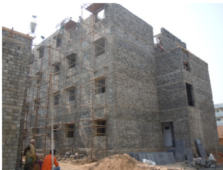
Figure 10. A Four storeyed housing with interlocking blocks at Vapi, Gujarat, India
