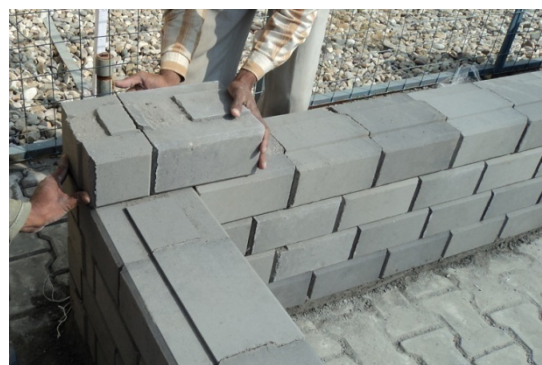
Figure 9. The corner masonry using interlocking blocks
