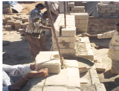
Figure 13. A Reinforced Masonry using interlocking blocks.
