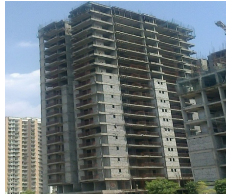
Figure 12. A multi-storeyed housing with interlocking blocks
