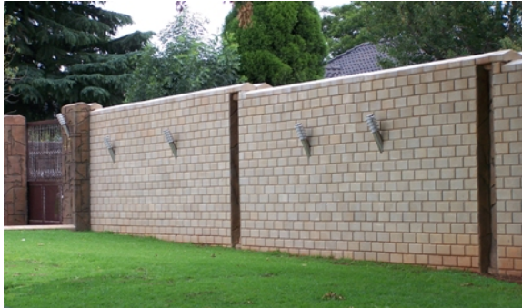
Figure 15. A boundary wall constructed with interlocking blocks
