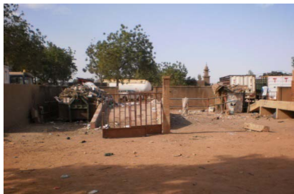
Figure 1. Example of waste collection infrastructure in Ouagadougou (2015)
