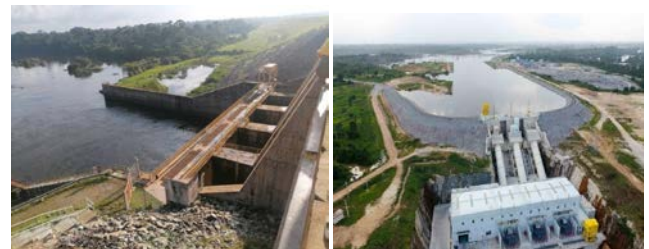
Figure 2. View of the Buyo dam (a) and the Soubré dam (b) on the Sassandra River [13]
