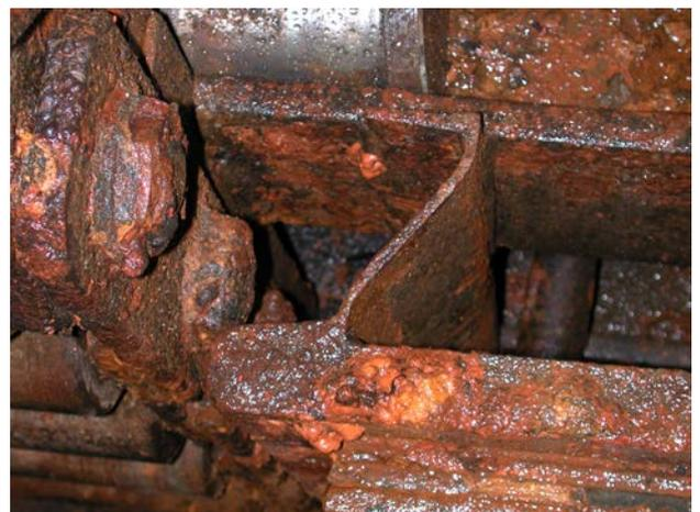
Figure 6. Corrosion of sluice gate structure
