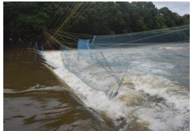
Figure 4. Checkdam fragmenting the river preventing fish migration
