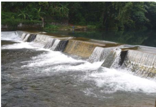
Figure 3. Check dam without fish passages
